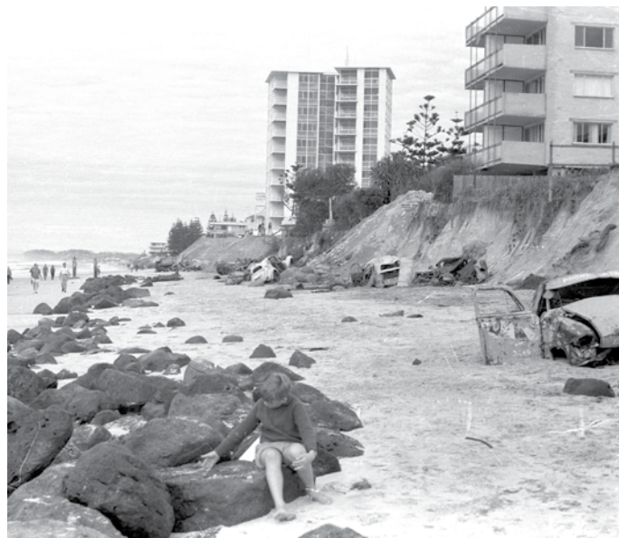
Car bodies and boulders were used to halt the progress of beach erosion on the Gold Coast, Queensland, 1967. Photographer unidentified. Gold Coast Libraries Local Studies Collection.
