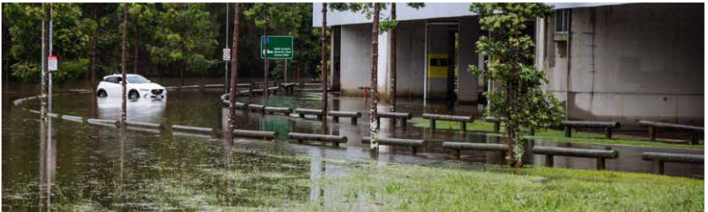
Flooding of low-lying areas
