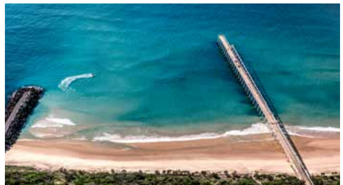
Gold Coast Waterways Sand Bypass Jetty, Gold Coast Seaway
