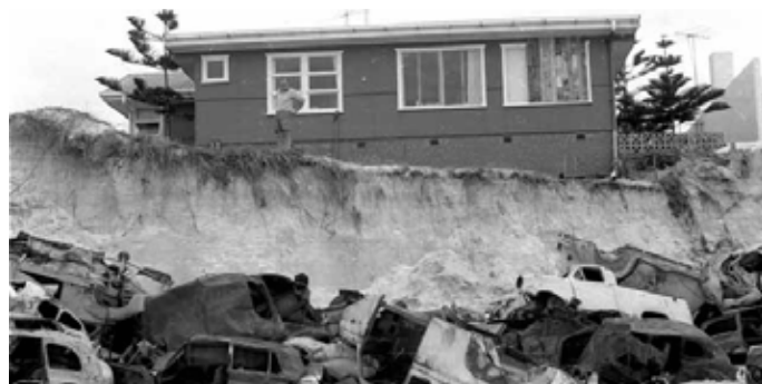
Car bodies used to try and stop the progress of beach erosion on the Gold Coast, Queensland, 1967. Photographer unidentified. Gold Coast Libraries Local Studies Collection.
