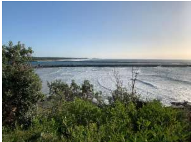
6 – Clarence River entrance breakwaters
