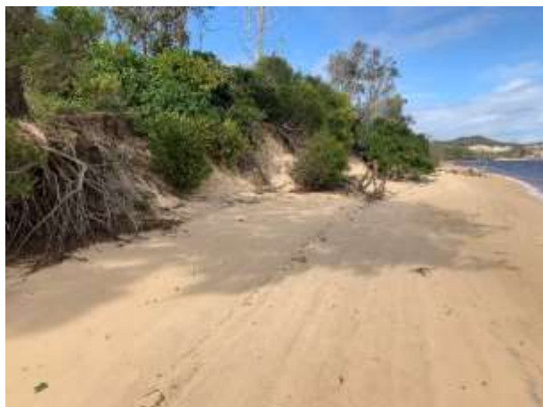
1 - erosion downstream of boat ramp
