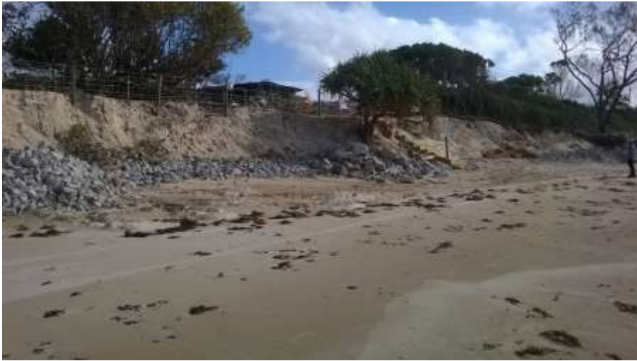
Plate 22: Beach erosion at Sandon river campground following the 2016 Black Nor'easter event
