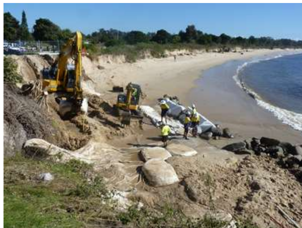
2 - Construction of GSC revetment
