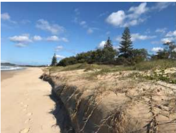
1 – Wooli Beach constructed dune
