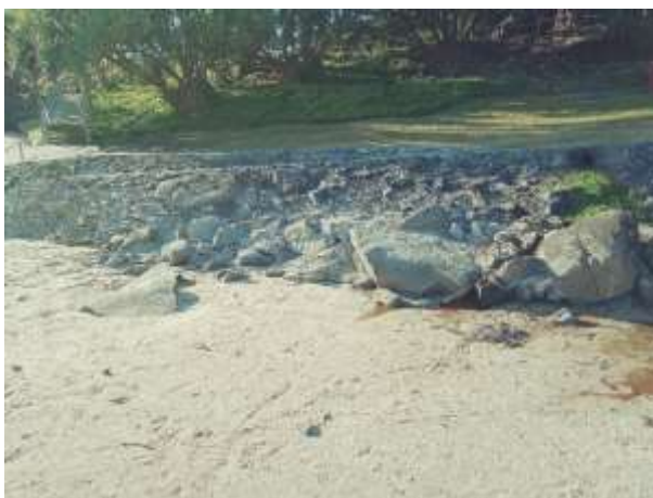
Plate 18: Yamba Main beach rock revetment
