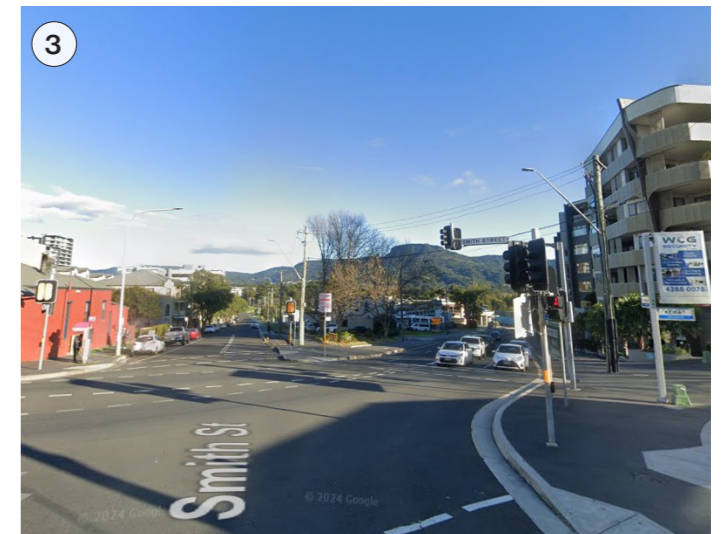
Existing view from Smith Street
