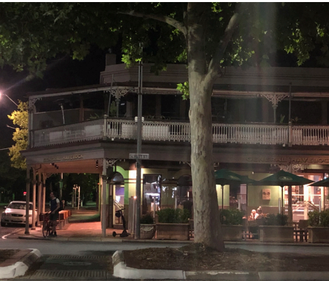
There are a number of opportunities to light façades of heritage façades
