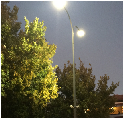
Goose-neck street lights in the median and at key intersections are outdated, glarey and not to a design quality representative of a main street environment
