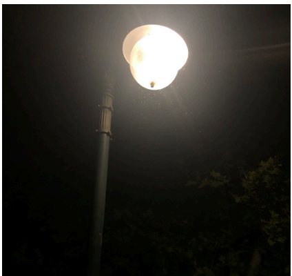
Metal halide lights (in faux-heritage posts) attract insects, creating maintenance issues and affecting the local ecosystem
