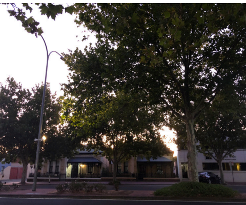
Some existing uplighting to tree canopies attached to goose-neck poles
