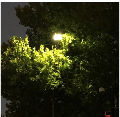
The tree canopies restrict the effectiveness of existing street lights and cast shadows
