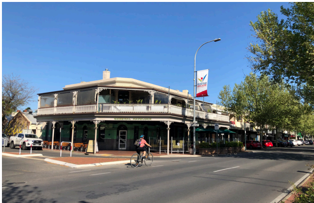
S5. 162-166 Hutt Street – General Havelock Hotel
