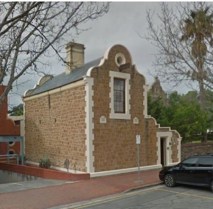
S1. 22 Hutt Street – Rymill House Coach House
