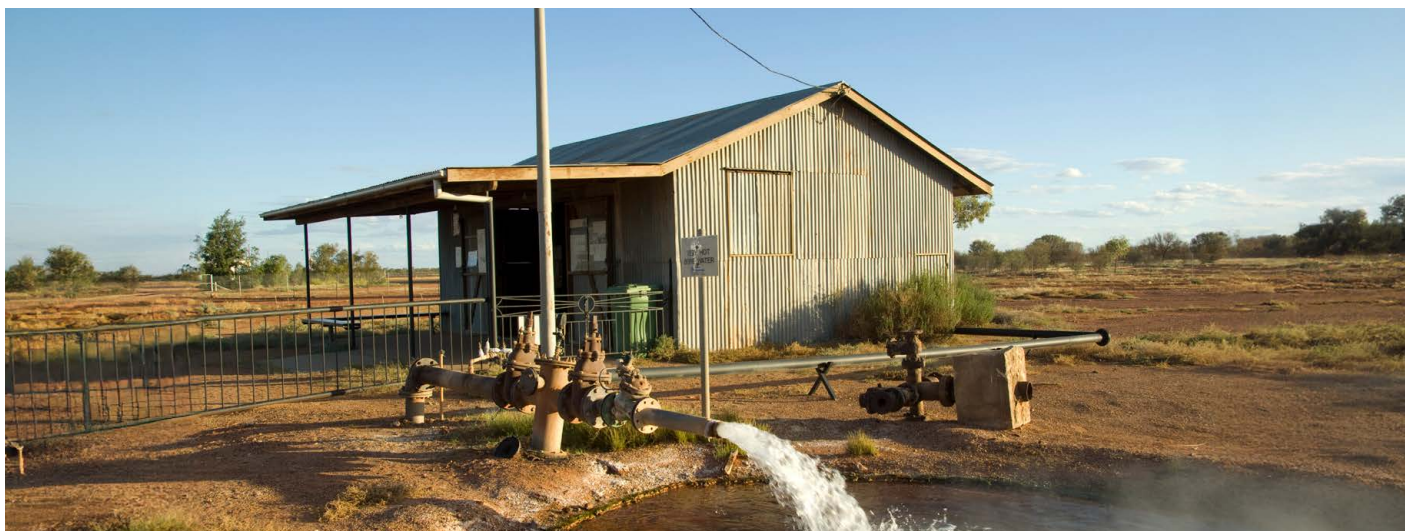
Borewater and pump, outback farm
