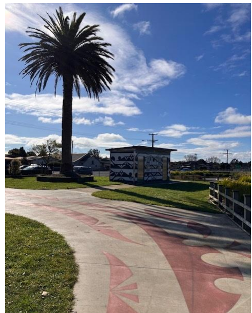
Figure 2320: Exeloo Toilets (Northern End)
