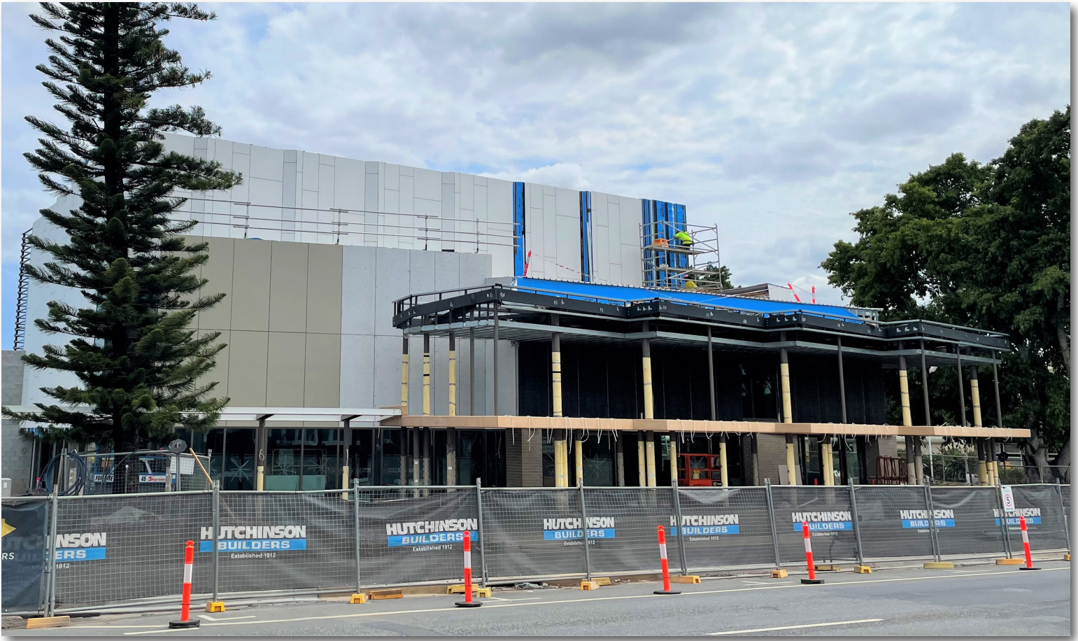
Proserpine Entertainment Centre construction in progress
