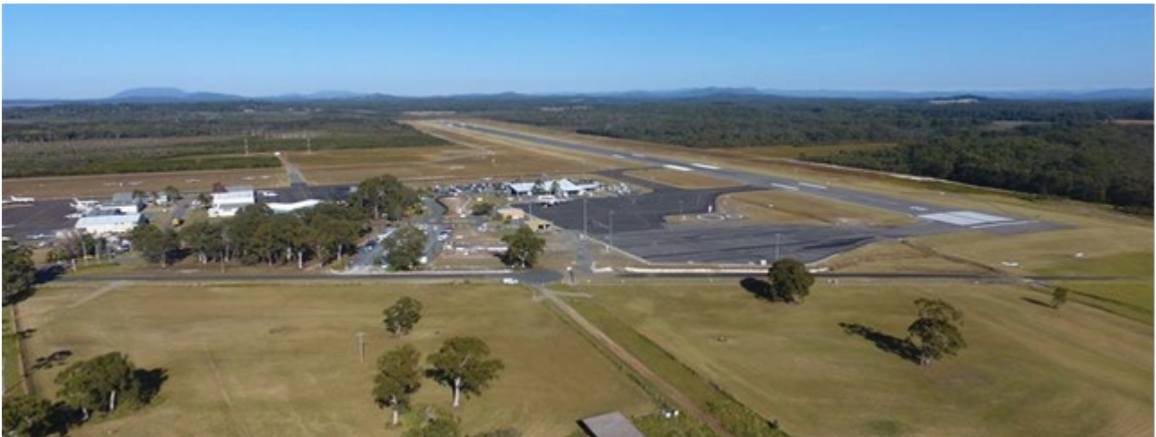
Figure 1: Aerial view of Port Macquarie Airport from the north (©Port Macquarie Airport)
