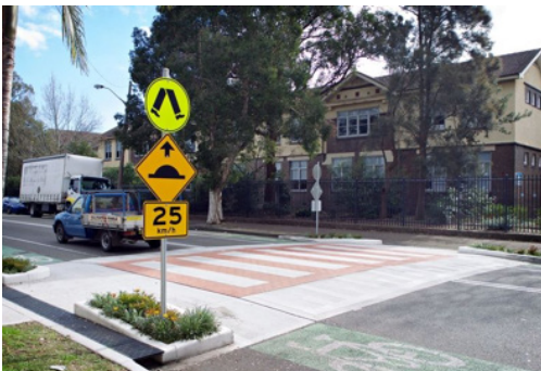
Raised pedestrian 'wombat' crossing
