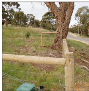
Figure 8. Fenceline strut arrangement. Note: this approach may not be appropriate for smaller trees, and an effort should be made to avoid structural roots when placing the post hole for the strut next to the tree.
