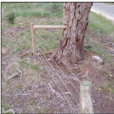
Figure 8. Fenceline strut arrangement. Note: this approach may not be appropriate for smaller trees, and an effort should be made to avoid structural roots when placing the post hole for the strut next to the tree.
