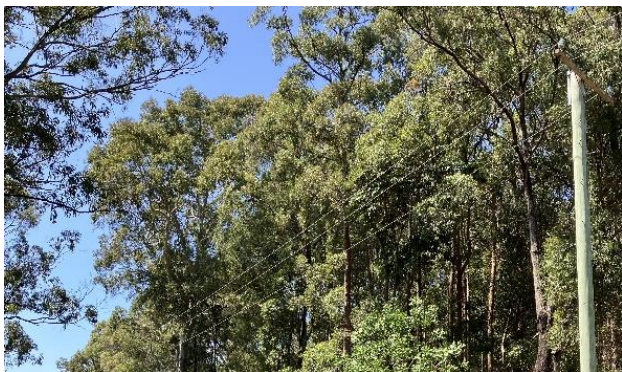
Examples of trees that may be removed or trimmed where the potential for damage to the network and bushfire risk is increased.
