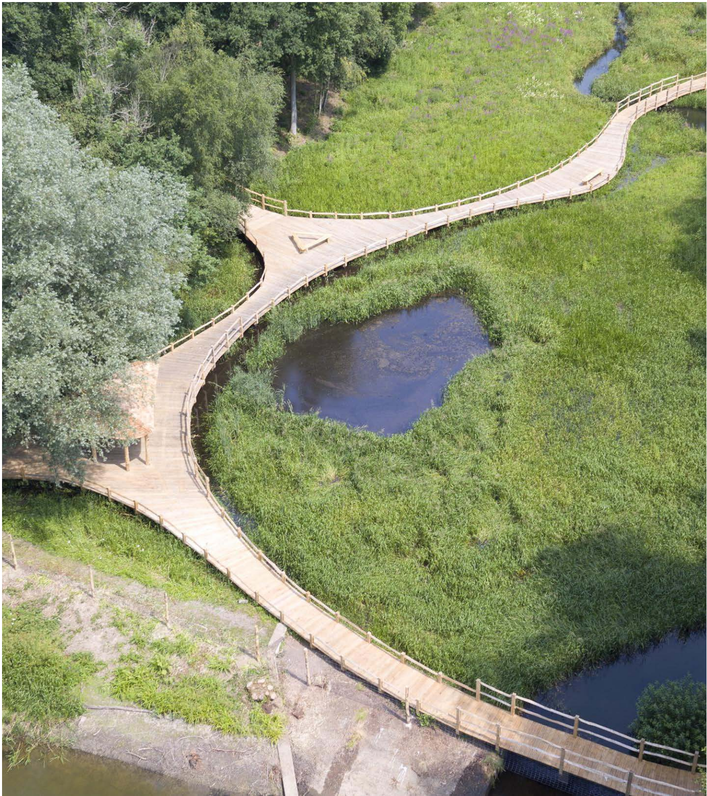
Boardwalks through wetlands and riparian areas
