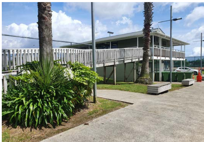
Buildings associated with the tennis club
