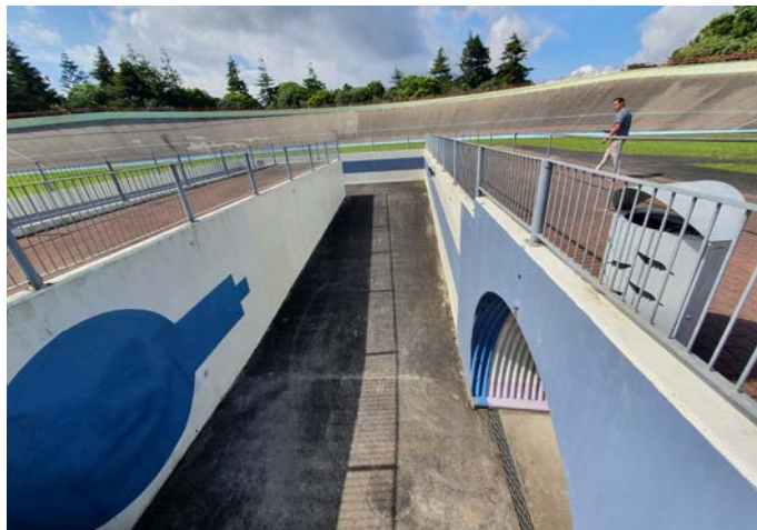
Cycle tunnel at the velodrome
