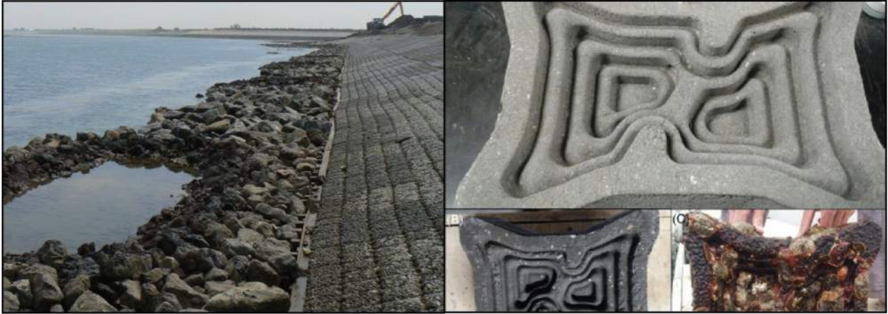
Figure 4-1: Photographs of “rich” revetment
