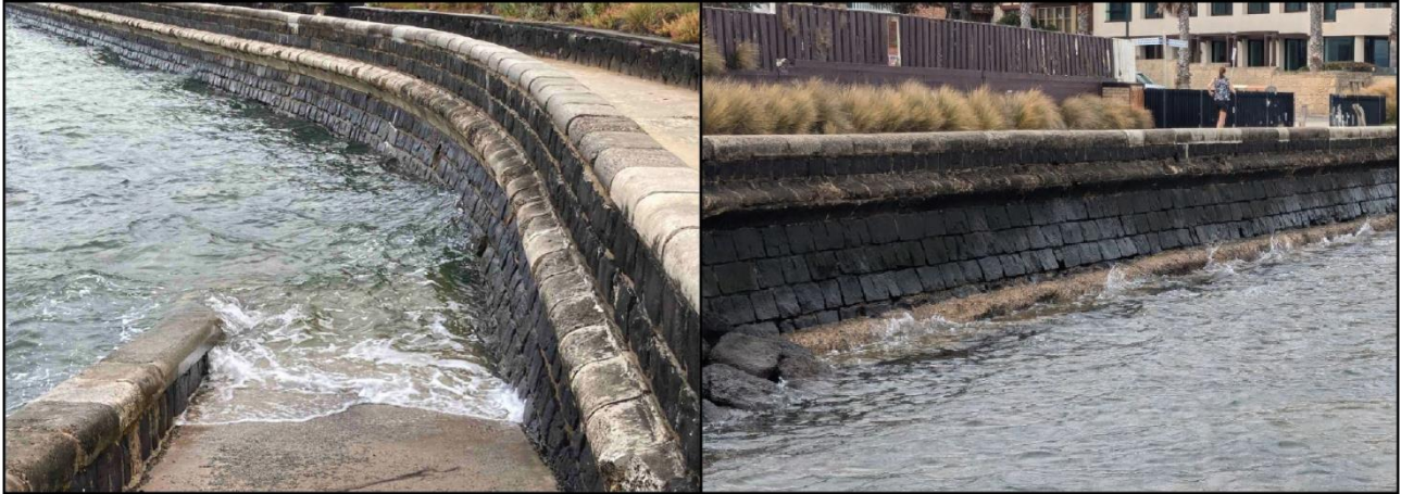
Figure 6-1: Photographs of vertical seawall
