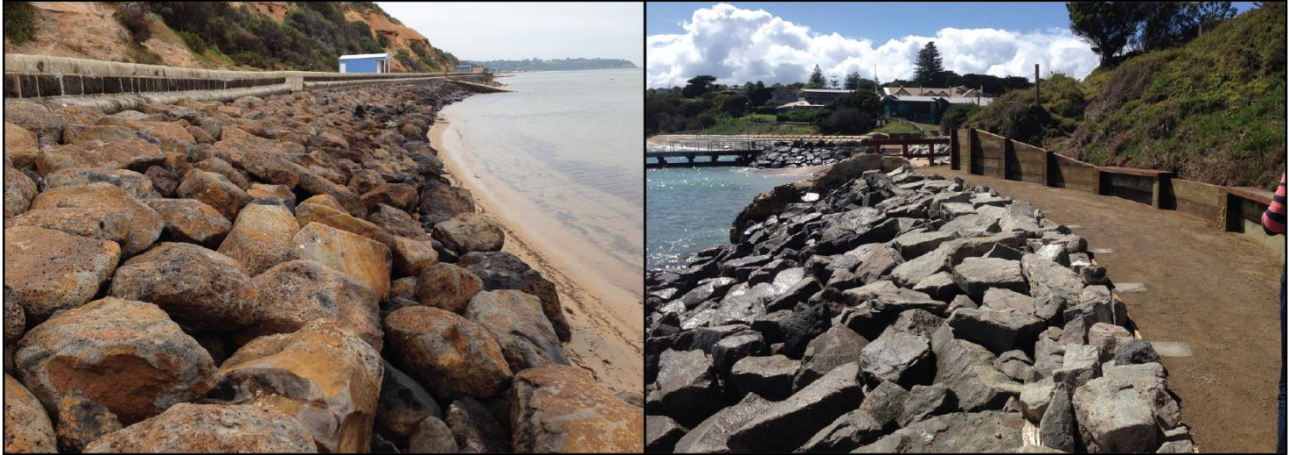
Figure 5-1: Photographs of rock revetment
