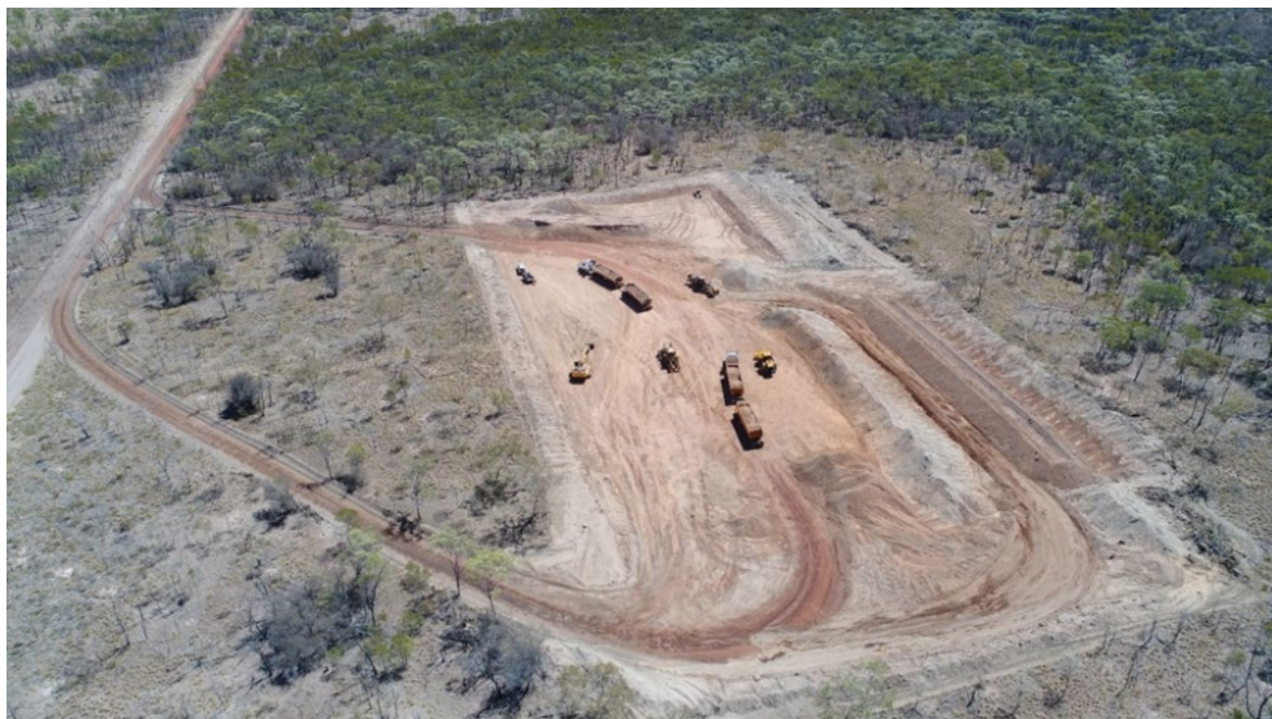
Figure 14: A typical operational gravel pit
