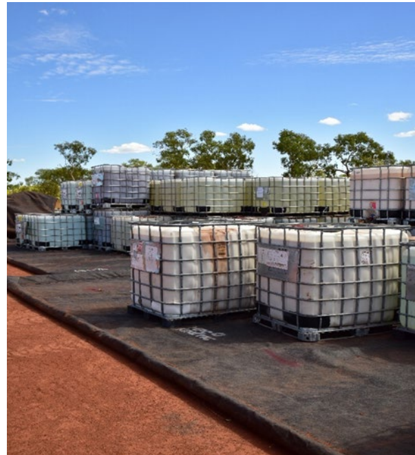
Figure 49: Examples of spill mats used to contain potential wastewater transfer spills
