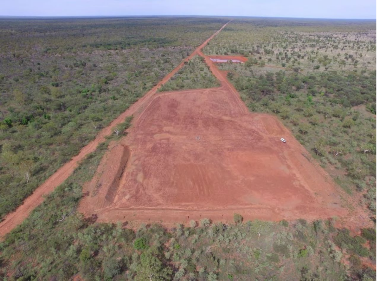
Figure 3: Existing Beetaloo W-1 disturbance footprint including lease pad upon which the approved Beetaloo W-1 stratigraphic well and associated activities are located
