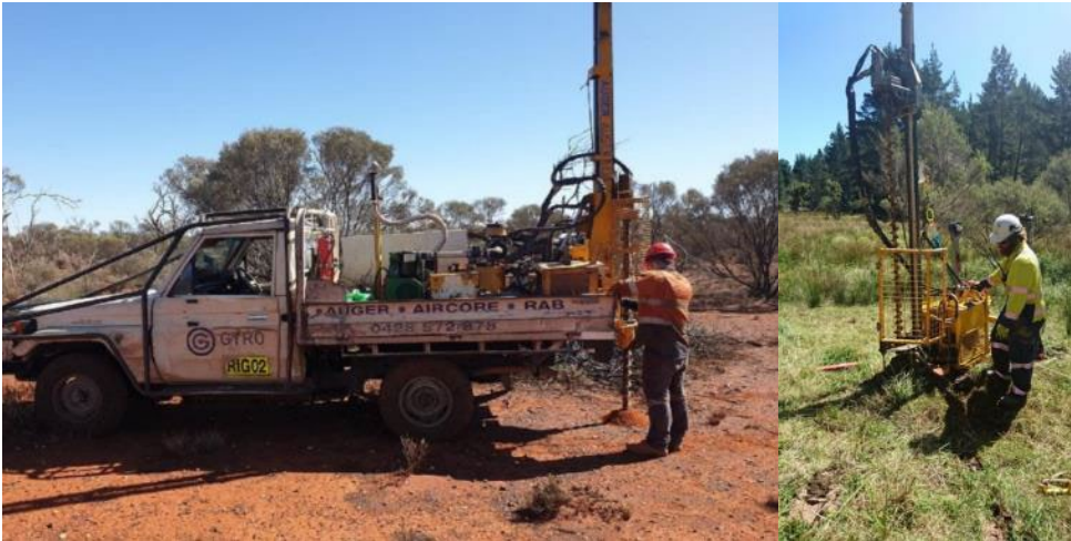
Figure 9: Example of a small rig that could be used for installing dynamite charges during a seismic survey
