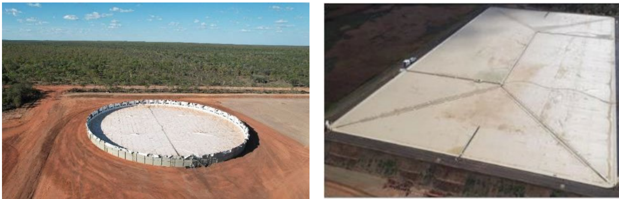
Figure 26: Examples of covered wastewater tanks used across Tamboran's sites (Riptide left; Flexipond right)
