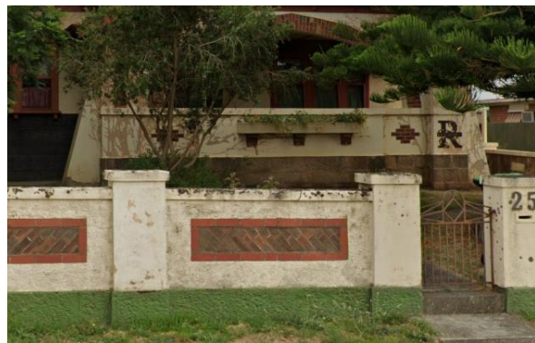
Figure 33. Detail view of bluestone base at 25 Barkly Street, Maryborough derived from the former Maryborough Gaol buildings.
