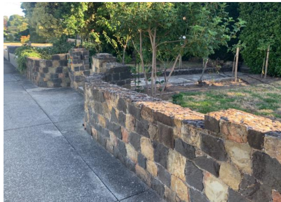
Figure 16. Bluestone and sandstone block front wall at 100 Inkerman Street, Maryborough.
