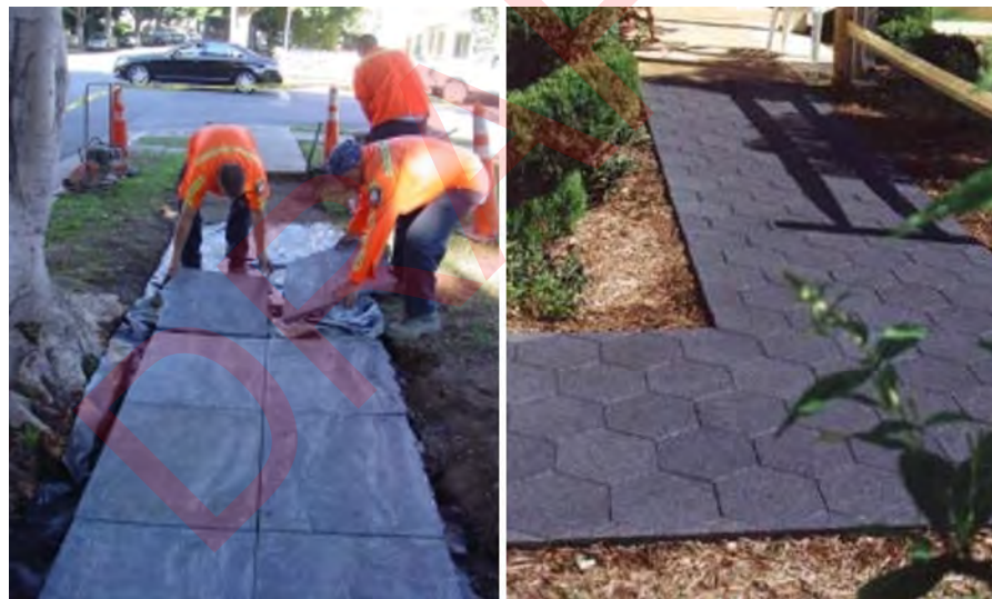
Figure 4: Installation of rubber paving (L) and a finished path (R).
